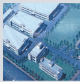
Wuxi Plant (China)
